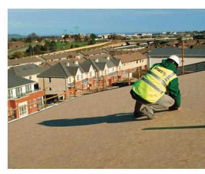
• Non-bracing sarking (non-structural): For a particular set of conditions, defined in terms of design, load and environmental conditions, long-term experience has demonstrated compliance of the design with specified requirements. These designs are "deemed to satisfy" and Table 2 (below), which is extracted from 'Panel Guide', provides the minimum thickness of OSB at certain support centres and is based on long-term experience:
