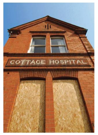
**Suitability:** EN 300 classifies OSB panels by their properties which relate to their intended use. SmartPly OSB2 is classified as a load-bearing panel for use in dry conditions.
